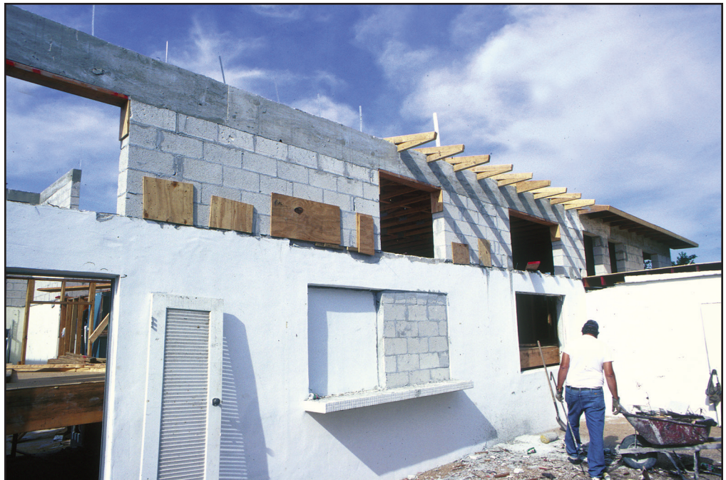
Figure 67 The extended first-story walls.
