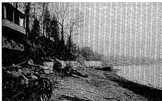
Erosion of bluffs overlooking the Great Lakes has caused an immediate hazard to many lakefront homes. Some were certified as being in danger of imminent collapse and were eligible for federal assistance under Upton-Jones to be relocated.
