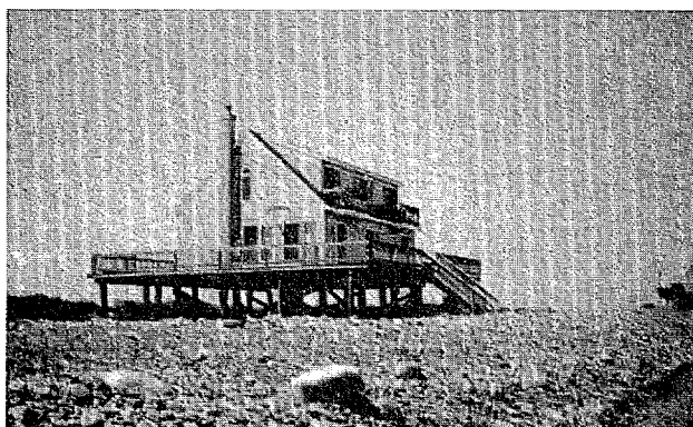
Decking is generally supported by concrete columns. Additional piles or a deeper foundation are used when disturbed soil is encountered.
