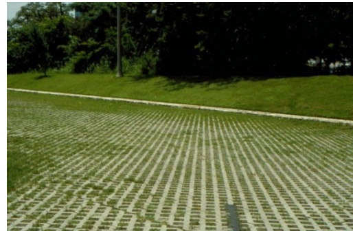
Figure 10-4.4.3-1: Example of Pervious Pavers
